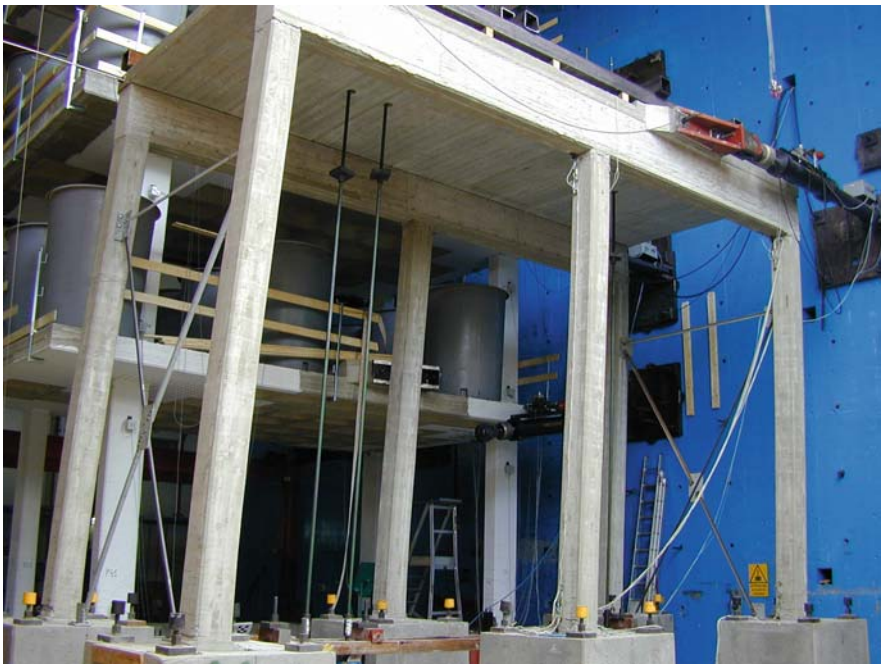
Fig. 10.13 Cast-in-situ mock up for pseudodynamic testing designed and built for the “Ecoleader” research project
