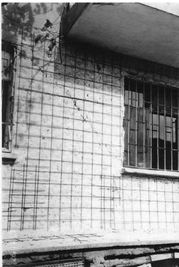
Fig. 8.24 Application of web reinforcement
