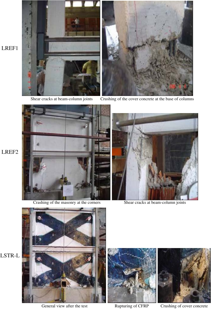
Fig. 18.5 Failure pattern of the test specimens
