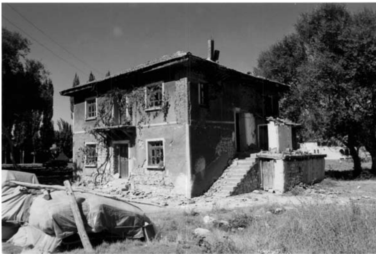
Fig. 8.7 Substandard plaster
