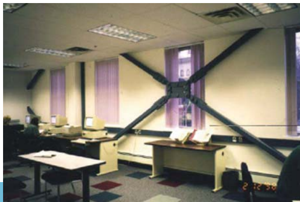
Fig. 6.12 X-braced friction damper in Harry Stevens Building
