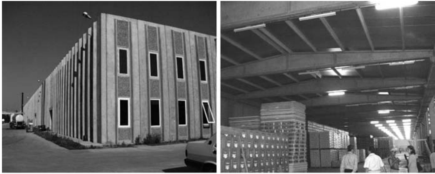
Fig. 9.5 Photographs of prototype building
