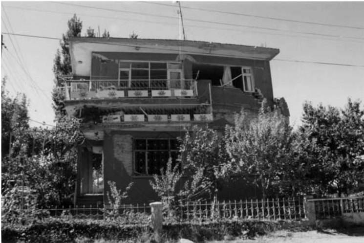
Fig. 8.13 Large openings in the walls
