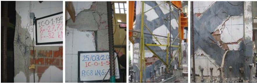
Plate 43 Some of the observed damages (see also Fig. 19.29 on page 407)
