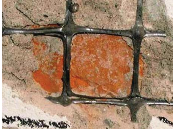
Fig. 6.11 Polymeric grids applied to masonry wall
