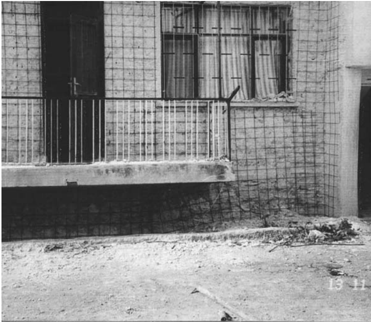
Fig. 8.25 Application of web reinforcement
