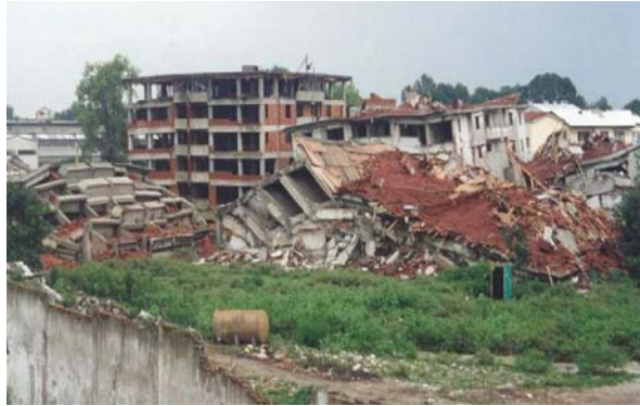
Fig. 19.3 Total collapse of low cost–low-rise reinforced concrete buildings (See also Plate 28 in Color Plate Section on page 471)
