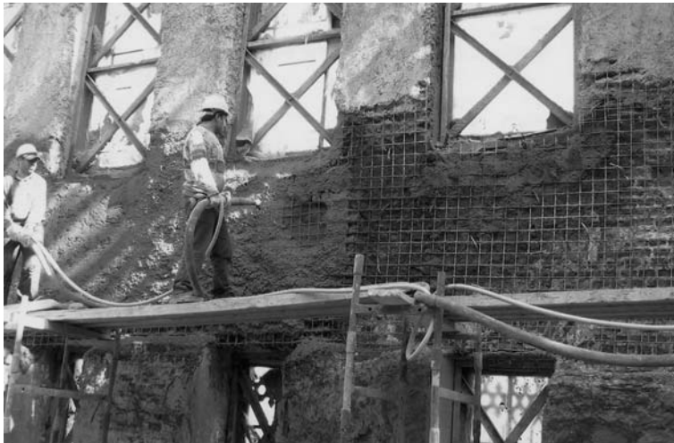
Fig. 8.26 Application of shotcrete
