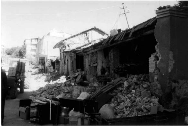
Fig. 8.6 Substandard wall units
